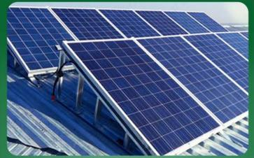
**Transition to renewable energy** Installed panels: 222 pcs. Annual generating capacity: up to 240 MWh
